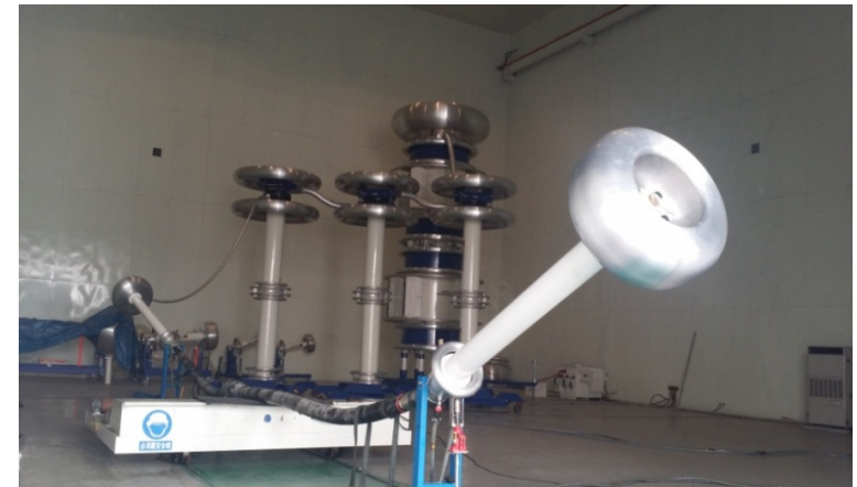
Experimental Setup for Electrical and Partial Discharge Measurement on 220kV PMJs
