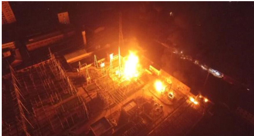
Fire in cable trench of 330kV substation, 18 June, Xi'an
